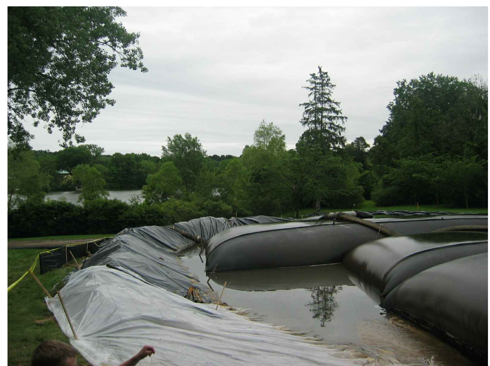
3 EXAMPLE GEOTUBE® CONTAINMENT AREA (HYDRAULIC DREDGING ONLY) NOT TO SCALE
